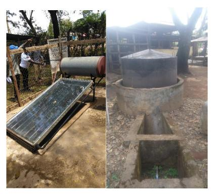
Plate 9- 10: Solar panel and a biogas digester
